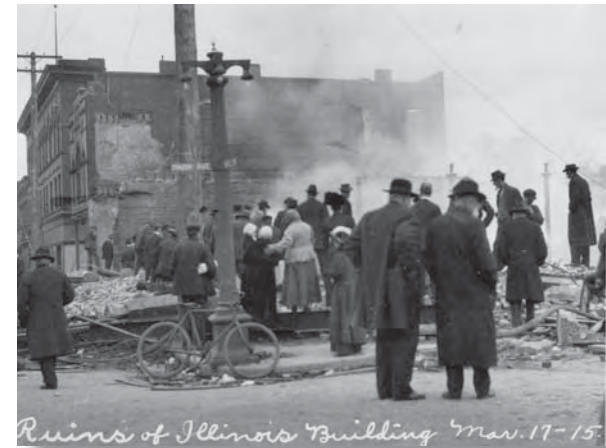
Ruins of Illinois Building Mar. 17-15. The St. Patrick's Day fire of 1915 destroyed the entire five story Lewis and Company Department store at the southwest corner Park and Neil Street. Fires like this were common throughout the early history of downtown.
