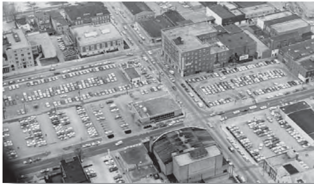
Over a 30 year time period over 60 buildings were leveled to make way for surface parking.. This movement did substantial damage to the urban fabric of downtown Champaign
