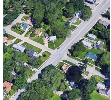
Existing intersection at Arcadia and Bellefontaine.
