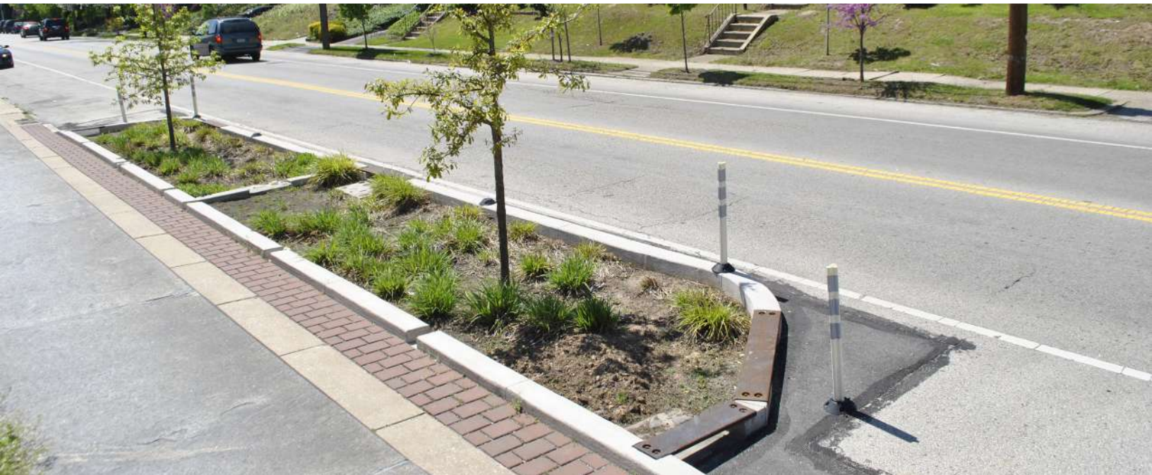
Bioswales can be incorporated into curb-bumpout designs.
