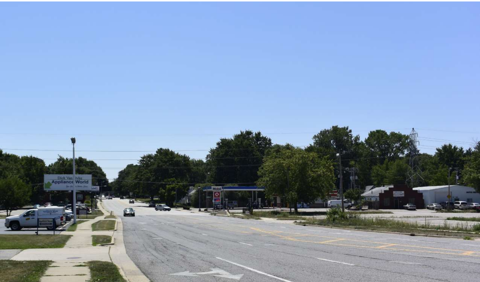
Existing view of the Neil Street Corridor near the I-74 Interchange.
