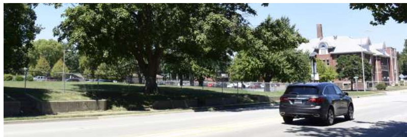
Existing retaining walls between Stratton Elementary School and Columbia Center.
